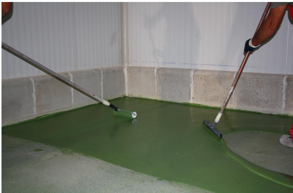
Aplicación de MAXURETHANE® CEM -S como capa de sellado antideslizante del sistema / Application of MAXURETHANE® CEM -S as anti-slip top-coating of the system
